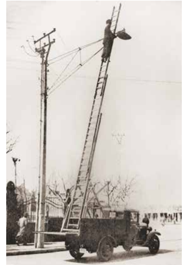
天津比商电车电灯公司员工安装电灯 CTET employees installing electric lights
