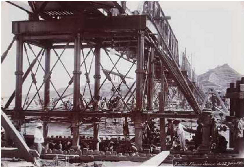
修建京汉铁路黄河大桥。摄于 20 世纪初（照片由比利时铁路公司某位职员拍摄，中国滨州窦希仑收藏） Construction of the bridge over the Yellow River for the Beijing-Hankou railway. Taken in the early of 20 century (Picture taken by an unknown Belgian member of staff at the railway company. Dou Xilun Collection, Binzhou, China)
