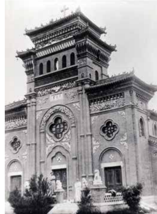
雷鸣远设计修建的河北省安国教堂，富于中西合璧风格 Vincent Lebbe designed and built the Anguo Church in Hebei Province
