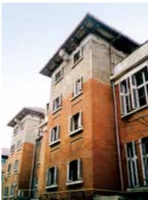
天津比商电车电灯公司职员公寓， 天津人称为“比国大院”， 约摄于 2004 年 The apartment building of the CTET staff, which is referred to as the "Belgian Compound" by Tianjin people, circa 2004
